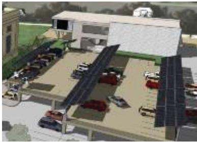
Solar panels on the parking and transit facility.
